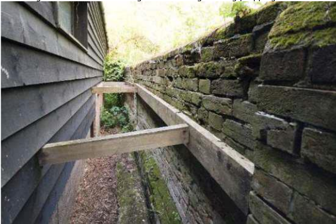
Figure 1 South wall curtilage lists showing existing propping
